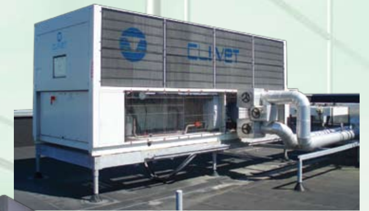
water chiller serving an AHU and fan coil units - 500kw cooling capacity
